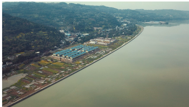
Figure 14. The impoundment of the flood control levee to an elevation of 335 m.
