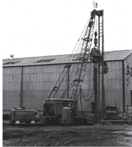
Figure 2. Sand compaction pile machine in the 1950s (courtesy of the Fudo Tetra Corporation).
