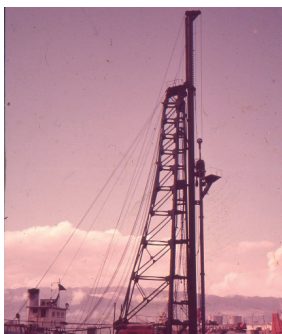
Figure 3. Deep mixing machine in the 1970s.
