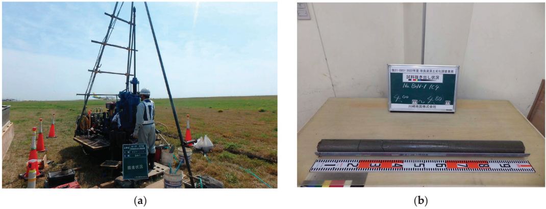
Figure 5. Boring and sampling: (a) boring operation; (b) core sample.
