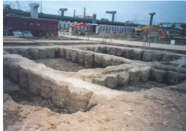
Figure 9. Grid-type DM-improved ground.
