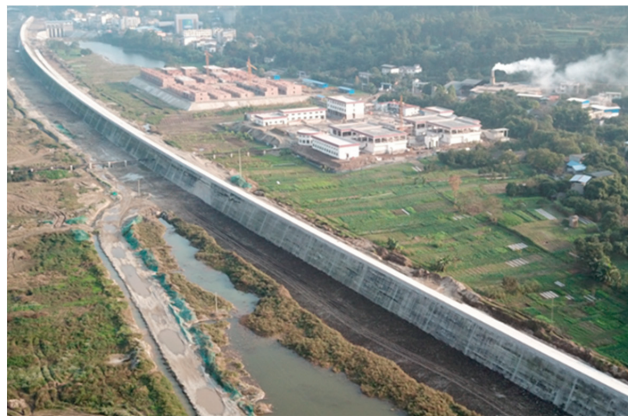
Figure 12. The completion of Tangba CSGR dam.
