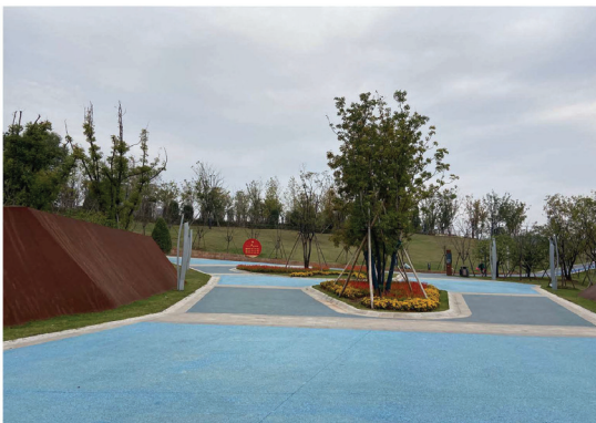
Pervious jogging trail added by sponge renovation project in Cuihu Park, Pingxiang
