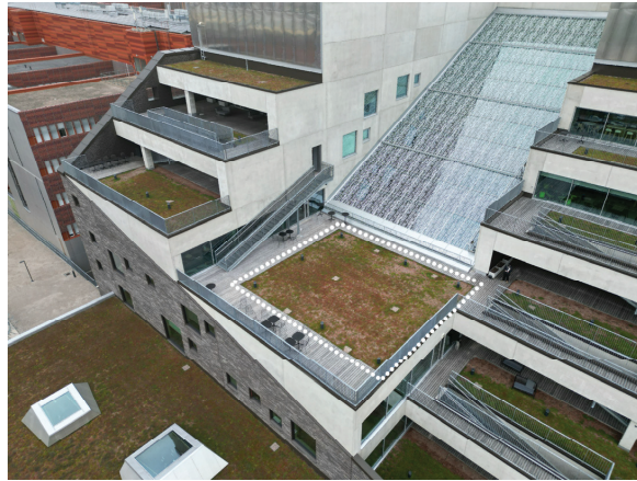
Figure 1. Demonstration site. The area subject to investigation is marked with a dotted line.
