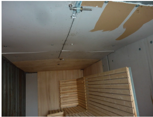
Figure 3. Test chamber: nozzles and heat detector.
