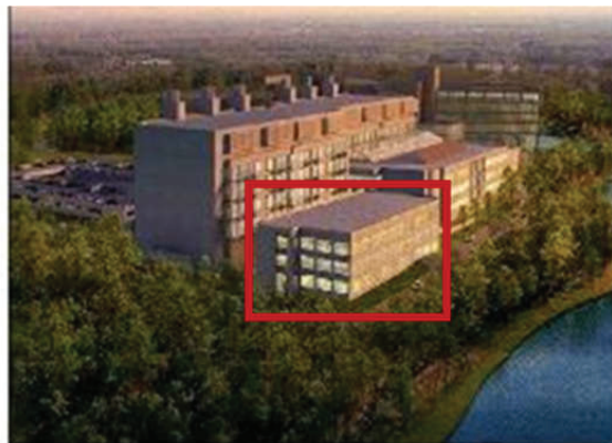
Figure 5. Overview of Target Building A.
