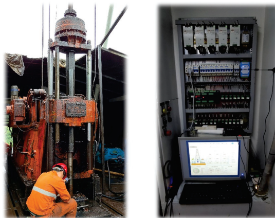
Figure 5. The drilling system of a real geological exploration well.
