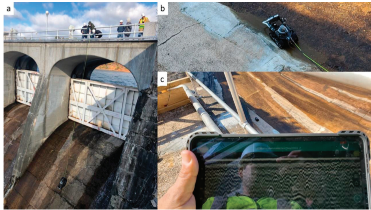
Figure 9. (a) Crawler with GPR being lowered onto spillway; (b) Crawler with GPR collecting data across repaired concrete surface; (c) Data collection with handheld device [82].
