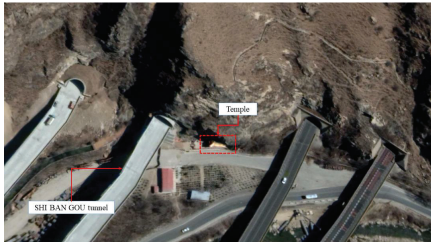
Figure 2. Route map of the tunnel (via Google Earth Pro).
