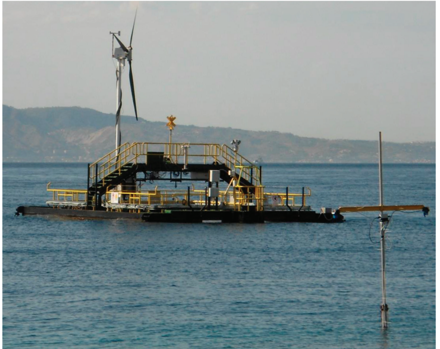
Figure 1. Photo of BGF platform installed at NOEL.
