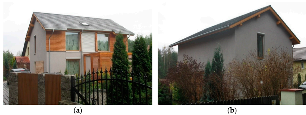
Figure 1. South-west facade (a) and south-east facade (b).
