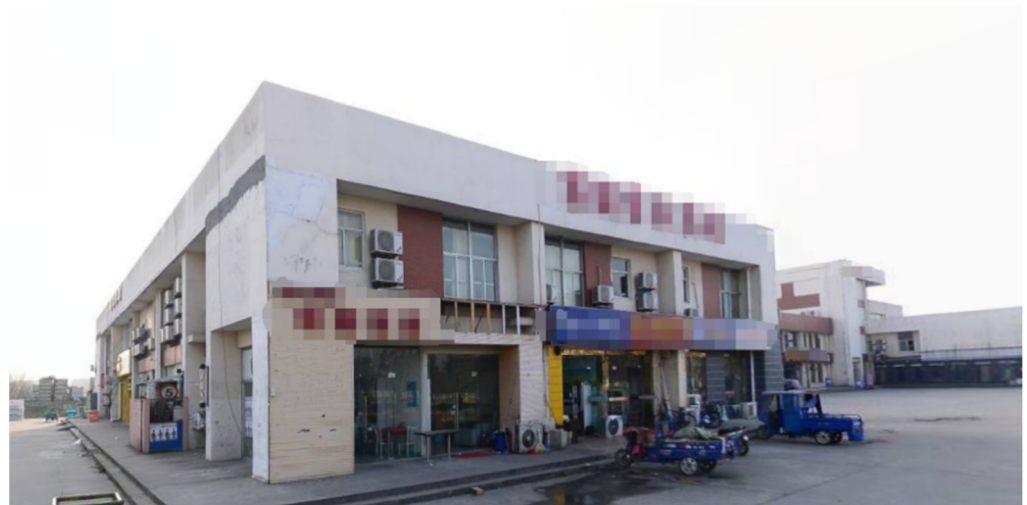
Figure 2. Measured 2-story building.
