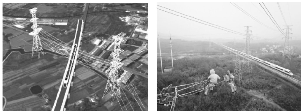
Figure 1. Cases of overhead transmission lines crossing high-speed railways.
