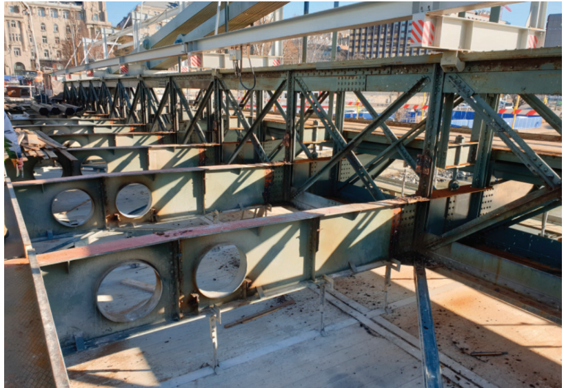
Figure 10. Superstructure with suspended scaffolding after demolishing old concrete deck.
