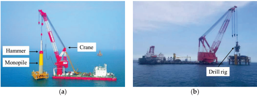
Figure 3. The on-site construction of: (a) monopile driving and (b) drilling rig hoisting.
