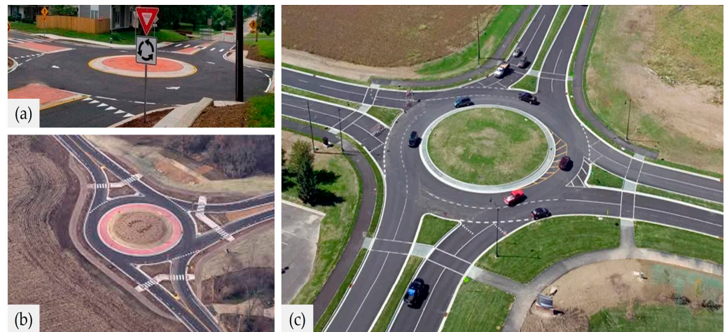
Figure 4. Basic types of roundabouts: (a) mini roundabout, (b) single-lane roundabout, and (c) multi-lane roundabout (with two lanes).
