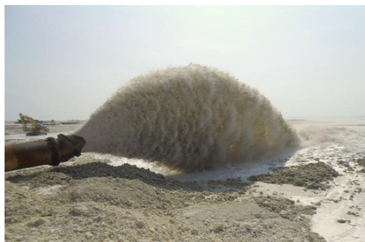
Figure 2. Formation of coral sand foundation.
