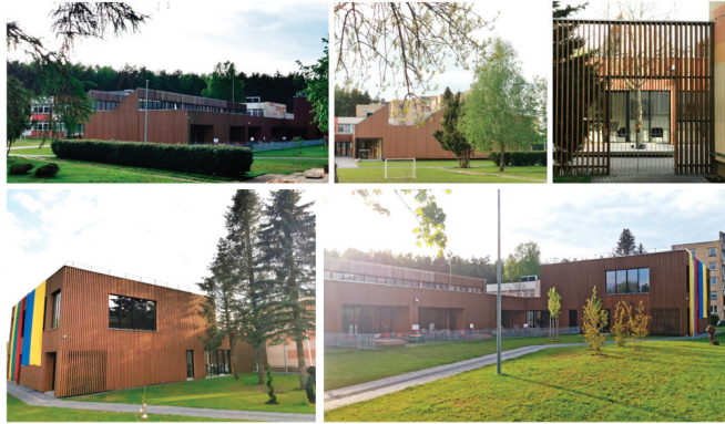
Figure 2. Kindergarten “Peledziukas” located in Vilnius, made with materials and roof configuration recalling traditional wood architecture was selected as an example of mimetic biophilic design. Photographs by A. Daugelaite.
