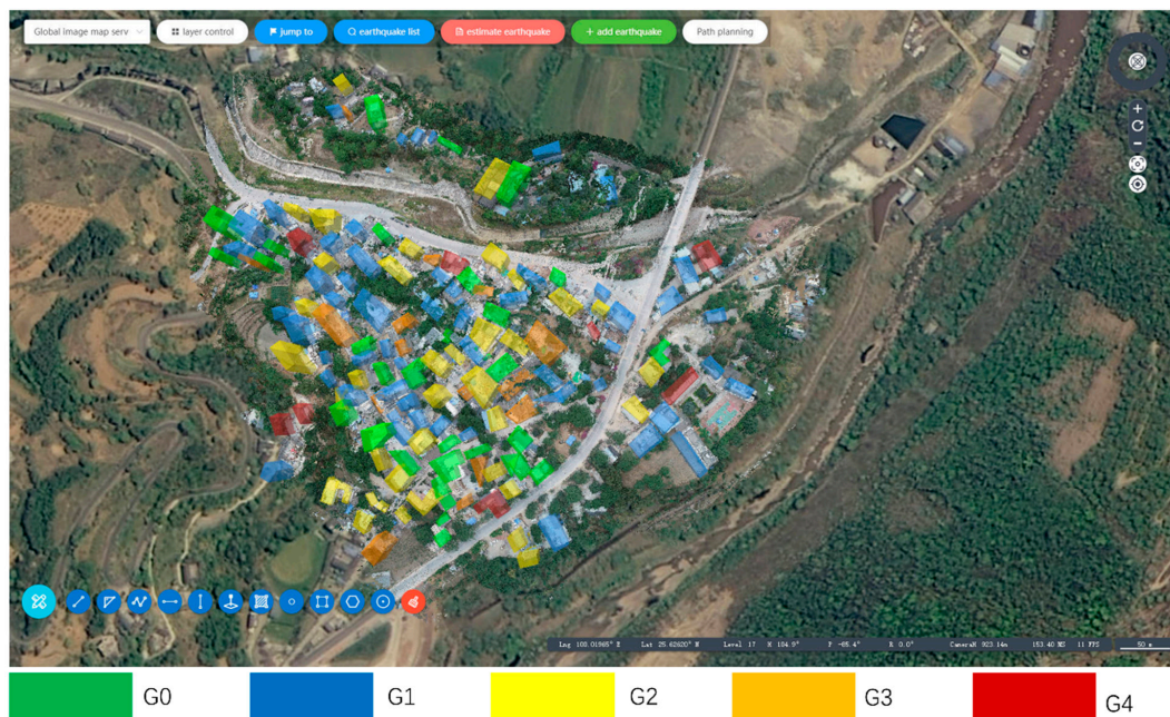
Figure 6. Results of the damaged assessment in Jinniu Village, Yangbi.
