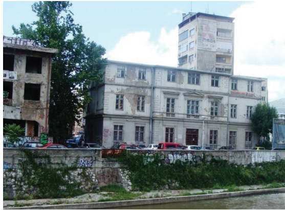
Figure 11. Hiseta administrative building before demolition of thermopower station on the left side (photo from 2015).
