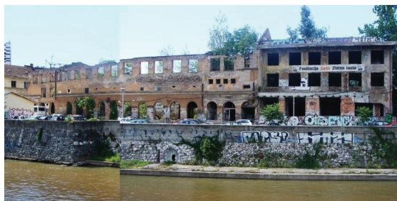
Figure 10. Hiseta thermopower station before demolition (photo from 2015).
