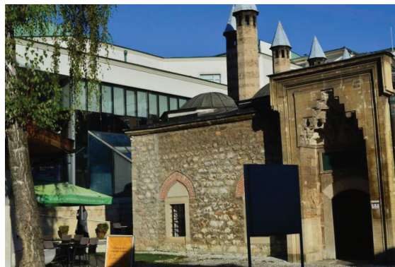
Figure 16. Gazi Husrev-beg Library—relationship with the historical building of Gazi Husrev-beg's madrasa.
