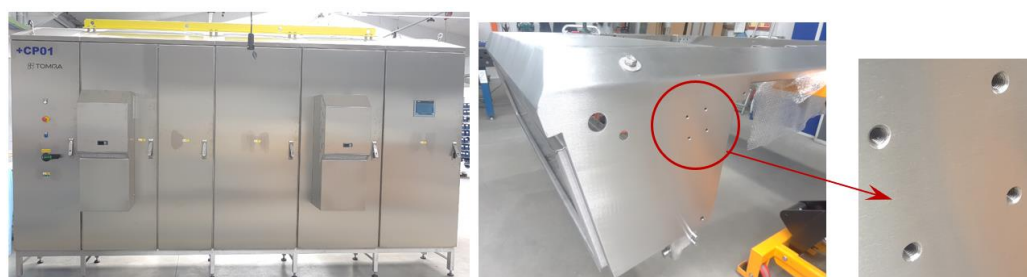
Figure 1. Electrical distribution cabinets monitored internal threads.
