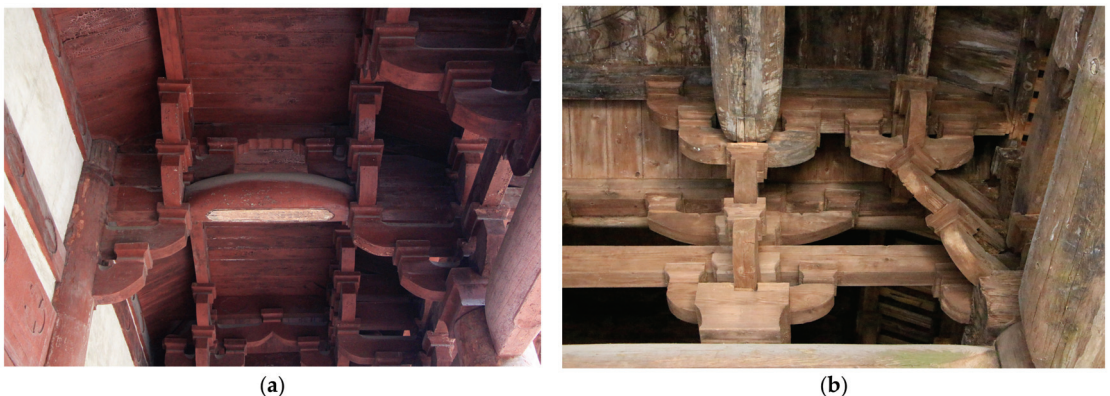
Figure 5. Clues for the form of palatial hall frames in eastern Fujian: beams intertwine with bracket sets to support the ceiling: (a) The front corridor of the main hall in Hualin temple; (b) the Song structure of Chen Taiwei Palace. Photography by authors.
