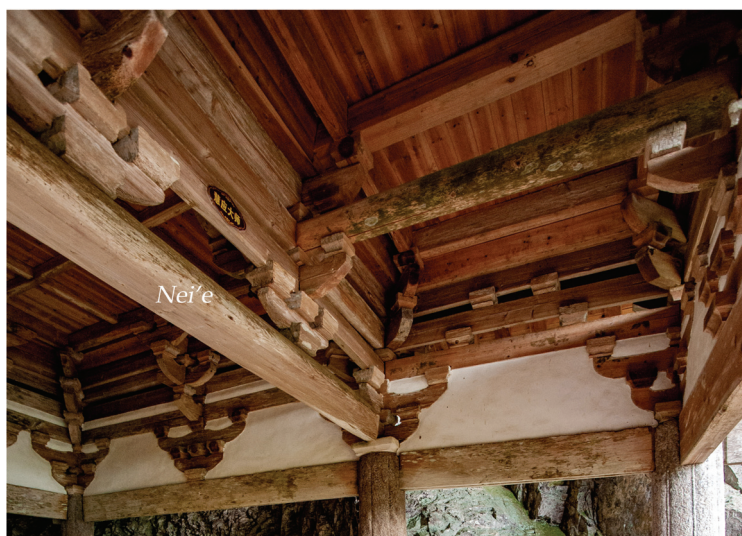
Figure 7. Internal longitudinal architrave connected with bracket sets to bear the beams in the Zushi Hall of Mingshan Temple in Yongtai. Photography by Xiaobin Li.
