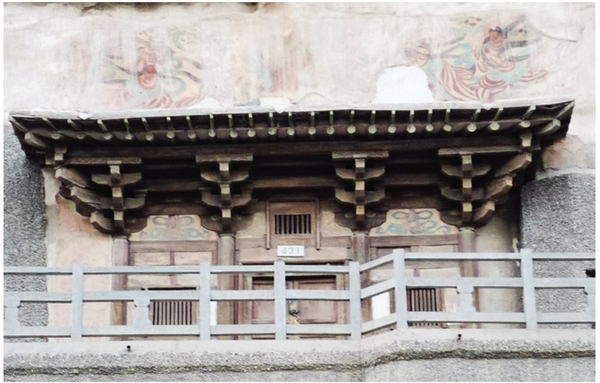
Figure 14. The timber-framed façade and exterior mural of Mogao Cave 431 showing three-step bracket sets, a three-bay façade, and an overhanging roof. Dated by inscription to 980 CE; 486 cm (w) × 142 cm (d) × 320 cm (h). Wood, mud brick, polychromic pigments. Photo by Zhenru Zhou, 20 January 2022.
