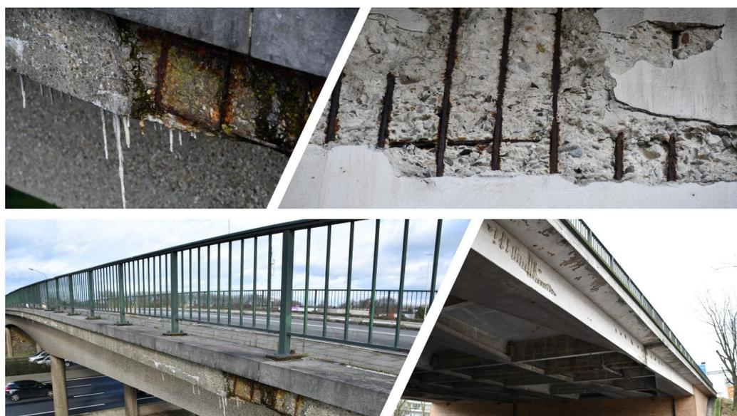
**Figure 1.** Examples of concrete spalling due to reinforcement corrosion.
