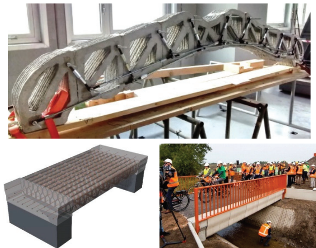
Figure 4. Meshed wires or cable implementation to C3DP bridge structures [102,103].
