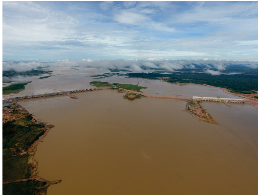
Figure 4. Aerial view of HPP Jirau. Right margin with 28 UGs on the left of the image. Left margin with 22 UGs on the right of the image.
