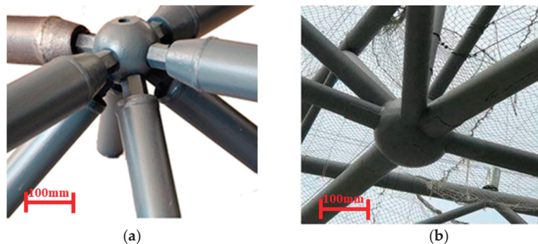
Figure 1. Typical joint types in space grid structures: (a) bolted spherical joint and (b) welded hollow spherical joint.
