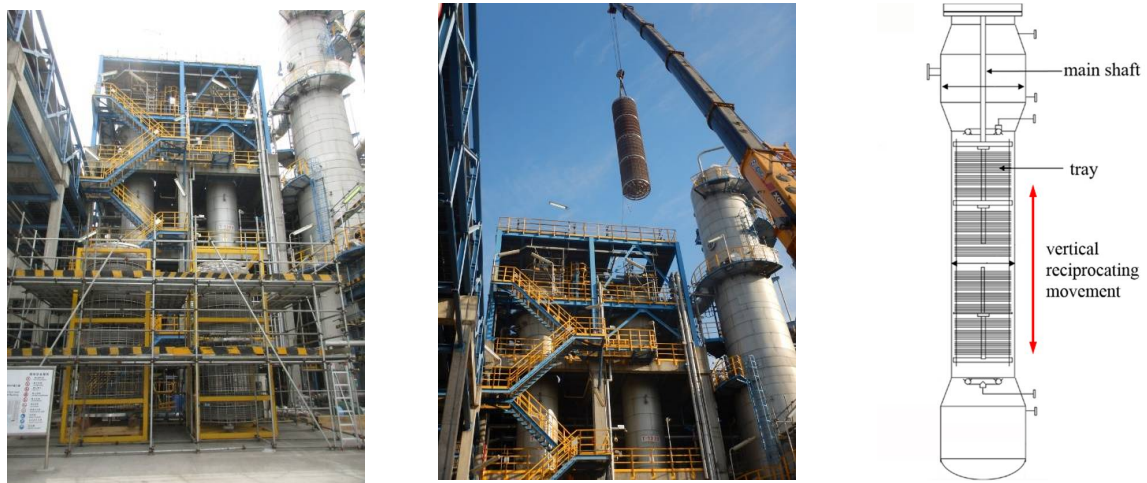
(a) in the vertical cylindrical shell shape (b) the tray pulled out from the shell (c) scheme of the tray and column
