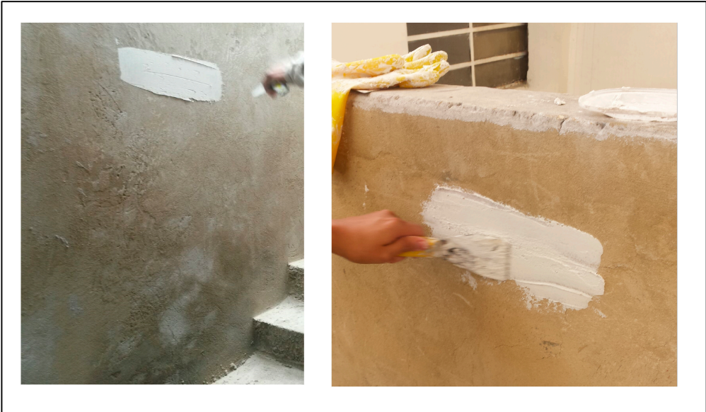
Figure 7. Detail of stucco application during indoor and outdoor performance tests.
