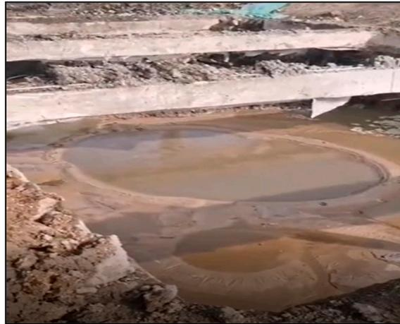
**Figure 11.** Water and sand gushing in the foundation pit.
