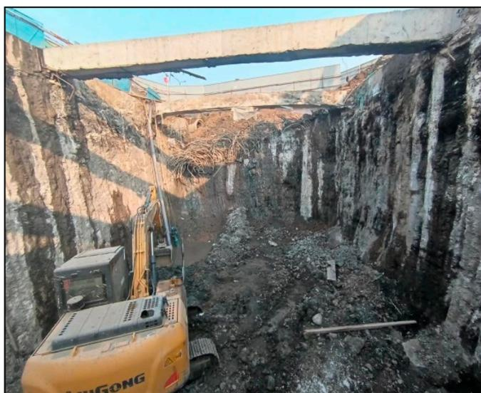
**Figure 14.** Excavation of foundation pit.
