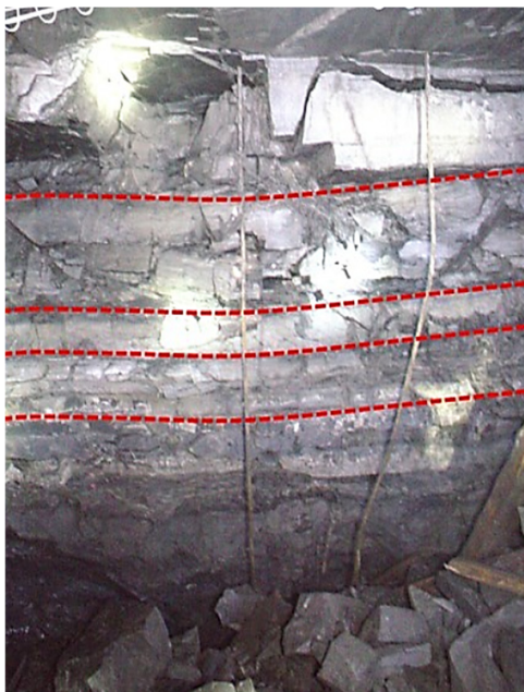
Figure 3. Composite Roof of Roadway Exposed On Site.
