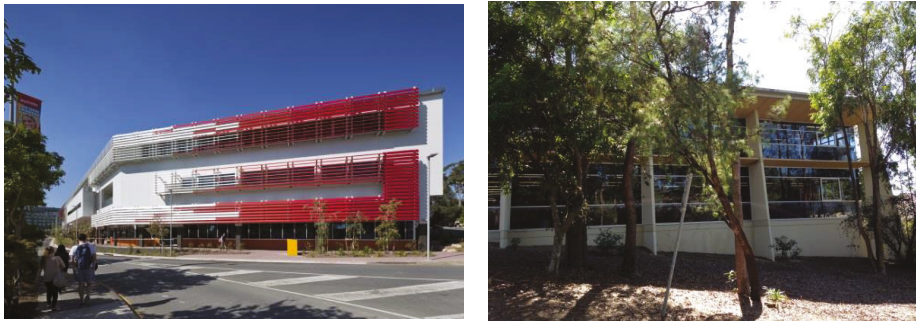
Figure 1. Griffith University Gold Coast Library and its shading strategies: louvers for west facing facades, horizontal and vertical projections for north, south and east facing facades, and trees around the building.
