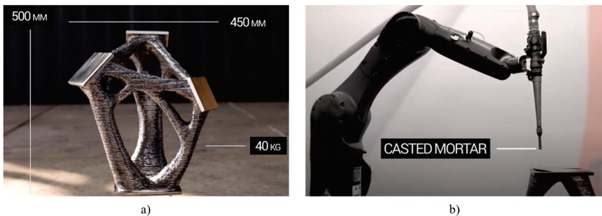
**Figure 19.** The Takenaka connector: (a) Geometry; (b) robotic arm filling the connector with casted mortar. Reprinted from ref. [123].
