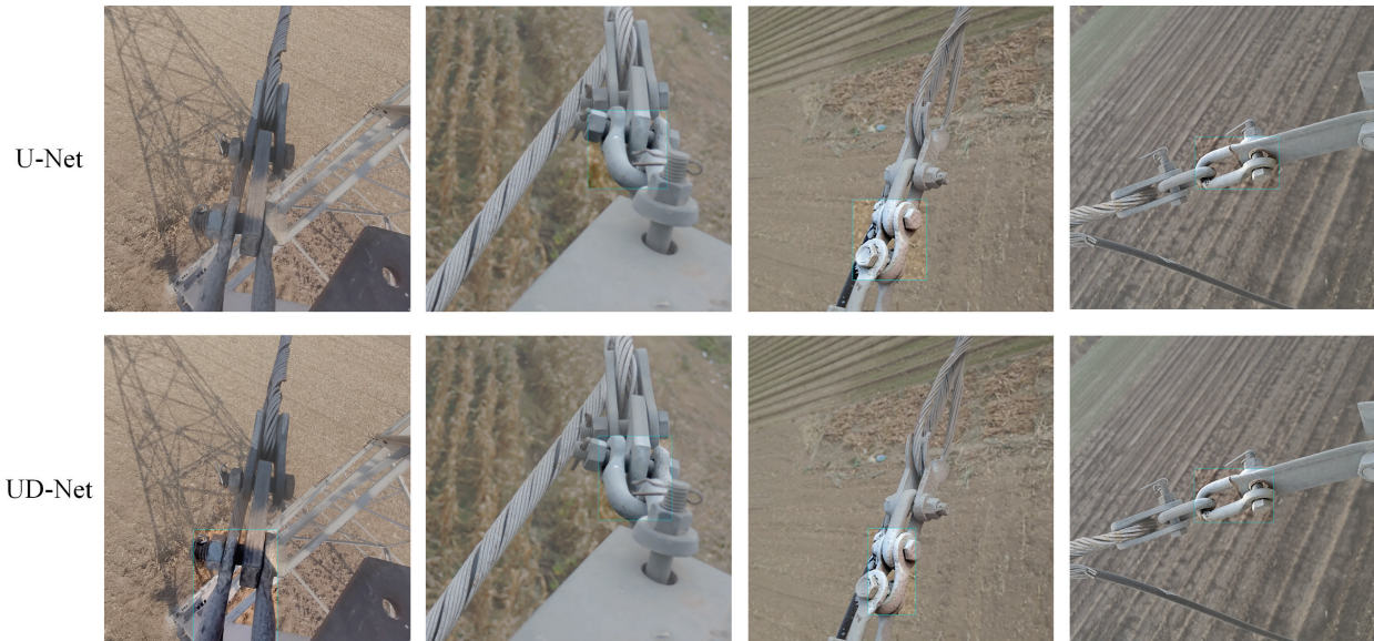
Figure 13. Visual detection results of shackles under yellow farmland scenes. The first row shows the detection results with U-Net and the second row displays the detection results with UD-Net.
