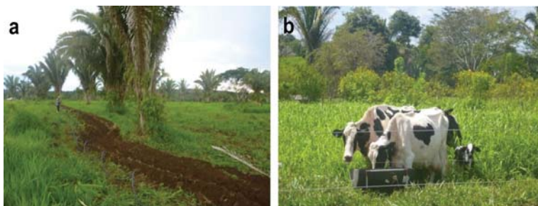
Figure 9. (a) Installation of underground piping to deliver water to each plot in the Silvopastoral System with Rotational Grazing for Dairy initiative; (b) Dairy cattle drinking from one of the water troughs, with electric fencing in the foreground.
