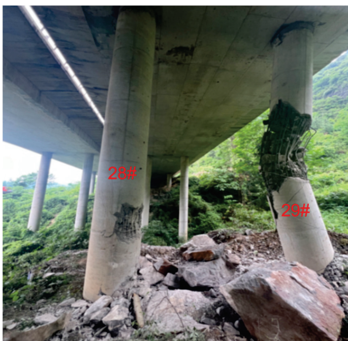
Figure 1. Disease conditions of pier columns 28 and 29 of Pier 2.
