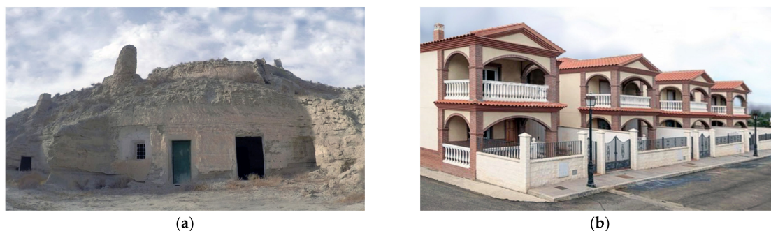
Figure 1. (a) Cave house in the Baza area. (b) Single-family houses in Guadix town. Source: own elaboration.
