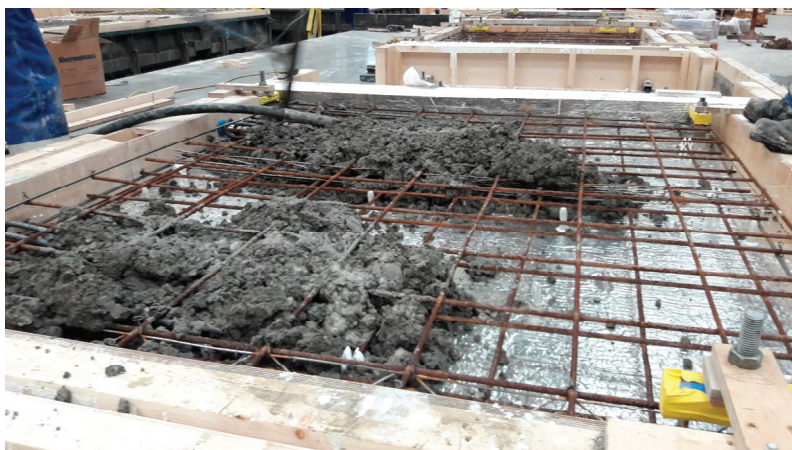
Figure 6. PCM-concrete composite panel under construction.
