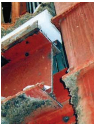
Figure 1. Steel structure damaged by Kobe earthquake in 1995 (reprinted from Ref. [1]).
