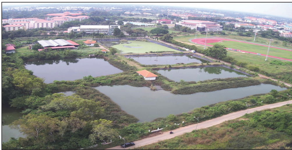
Figure 7. The sewage treatment system of Maharakham University.
