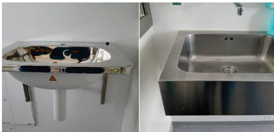
Figure 1. The self-disinfecting sink installed in room 1 is shown to the left, whereas the regular sink used in all of the other rooms in the Burn Centre is shown to the right.
