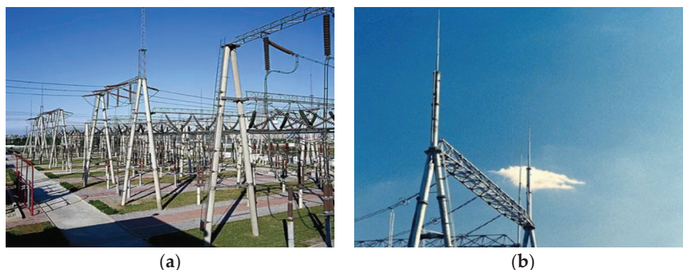
Figure 1. Substation structure and lightning rod structure. (a) A substation. (b) Frame–lightning rod structure.
