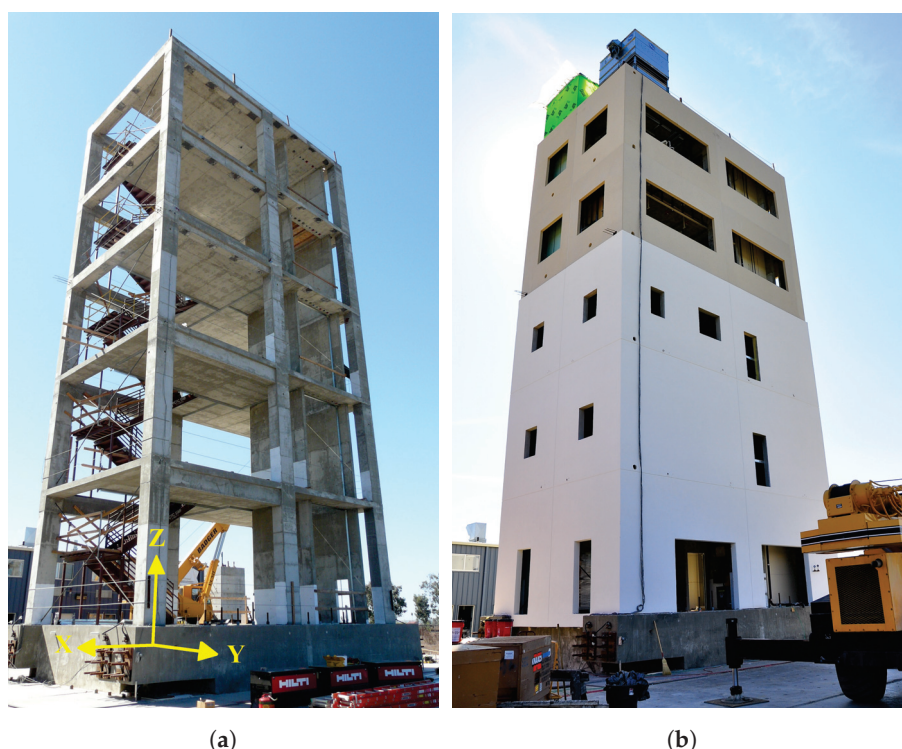
Figure 1. Five-story test building. (a) Bare structure without non-structural elements, (b) Complete structure.
