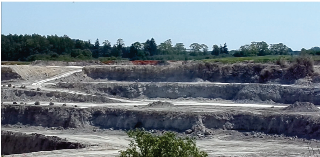
Figure 3. Blasting works at open-pit mine.
