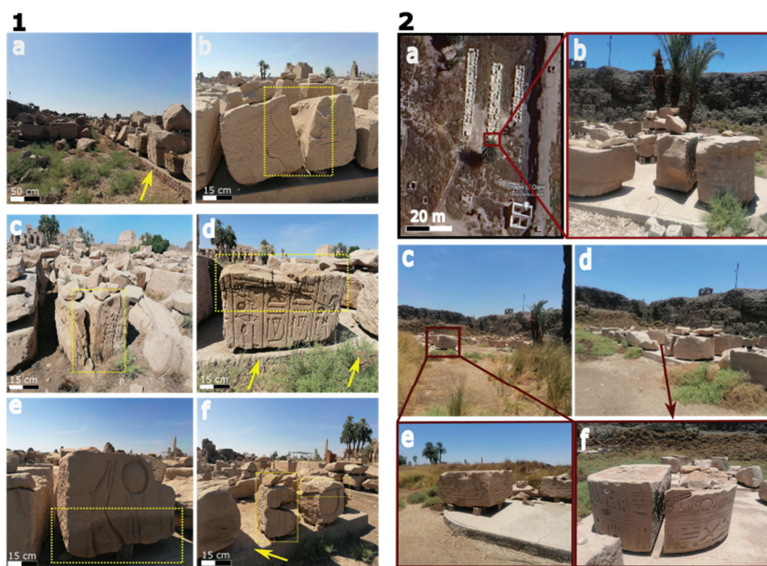
Figure 9. (1) and (2) Analysis of the mechanical impact of cumulative earthquakes and flooding events on the structures at Karnak. (1a) A general view showing scattered stone blocks, displaced due to mechanical forces, now resting on a loose red brick mastaba. (1b) Close-up of fractured stone blocks, illustrating the damage. (1c) Various stone blocks that have slid and become embedded in the soil, likely as a result of earthquake tremors or the impact of flooding waves. (1d–1f) Detailed views of mechanical chipping, fractures, and cracking observed on the stone surfaces, highlighting the extent of the damage. (2a) A Google Earth image of the study area, focusing on the northeastern part of Karnak, showing the current state of the stone blocks. (2b–2f) Documentation of various damage aspects of the stone blocks, including splitting, chipping, and fracturing, illustrating the ongoing deterioration of the site due to mechanical forces.
