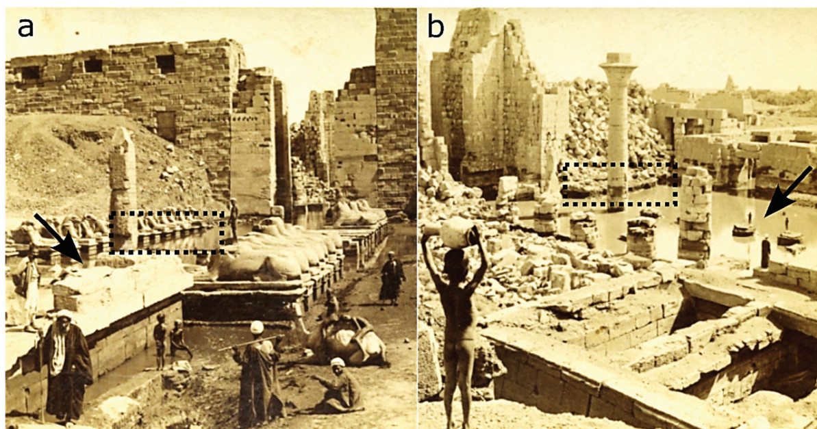
Figure 5. Two historical photographs from 1898 by B.W. Kilburn showing the first pylon of the Karnak Temples. The stone building materials are visibly affected by flash flooding, as indicated by black arrows and highlighted within dotted rectangles (a,b). From [59].
