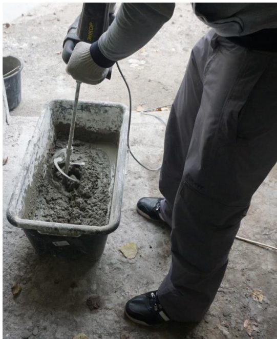
Figure 1. Mixing of the concrete mixture.
