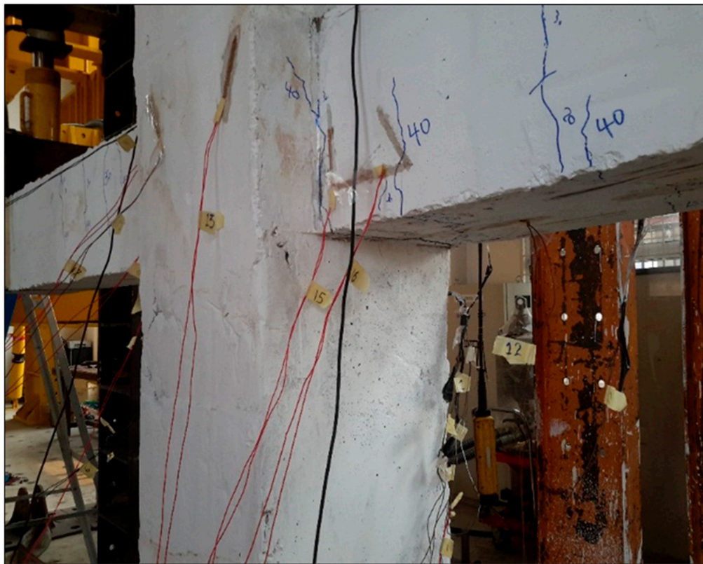
(a) Crack pattern in CS1
