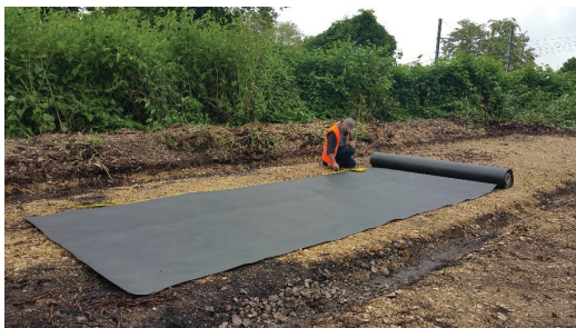
Figure 1. Installation of a synthetic geotextile as part of a tarping operation to control Asian knotweed. © INRAE.
