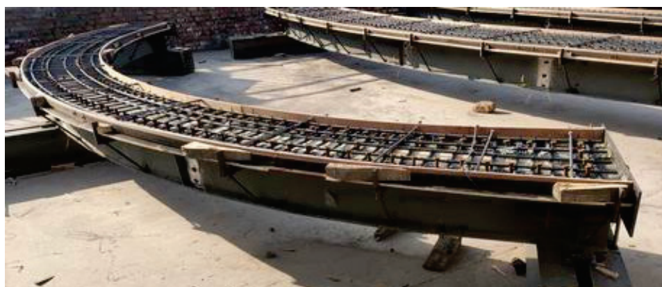
(c) Assembling reinforcement.
