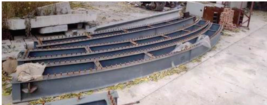
(a) Fabricated steel girders.
