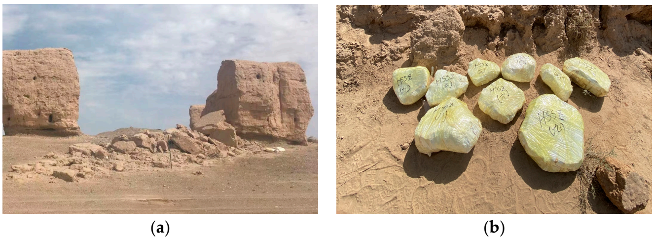
Figure 1. Crumbling earthen ruins and wrapped and packed soils. (a) Crumbling earthen ruins; (b) wrapped and packed soils.
