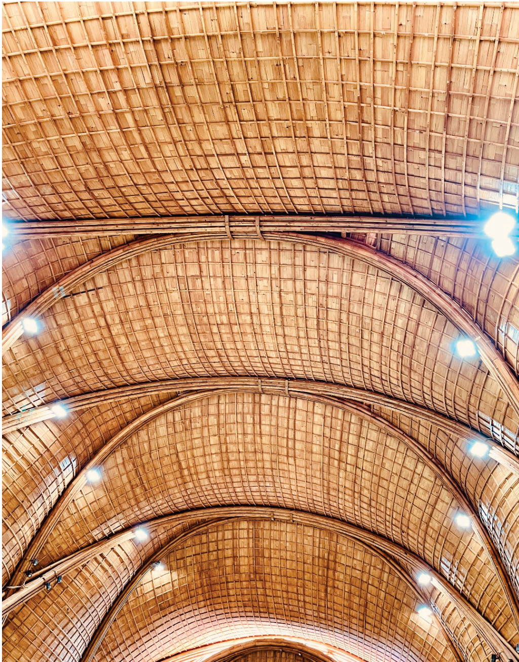
Figure 3. The rib-like structure of The Arc, designed by Ibuku (2021). Photo: Fiona Gray.
