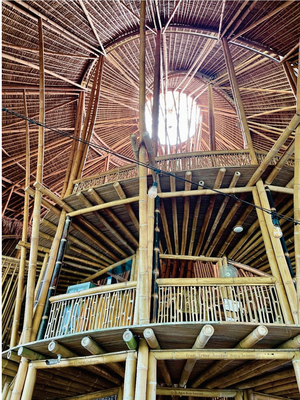
Figure 2. Towering bamboo columns supporting multi-level spaces of the Heart of the School. Photo: Fiona Gray.
