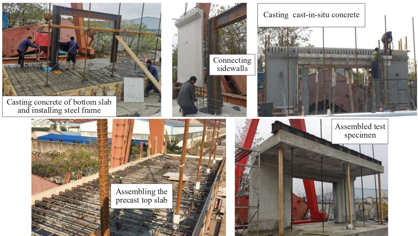
Figure 5. Construction process of the test specimen.
