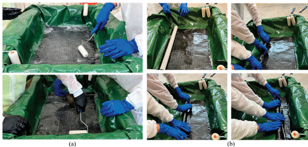
Figure 5. (a) Carbon fiber fabric wetting process for U-wrap. (b) Rolling wet fabric onto plastic pipe for layup on beam.
