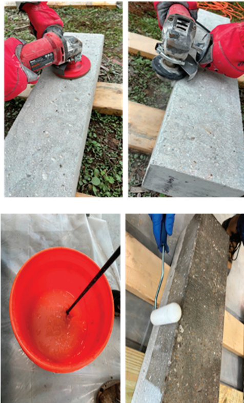
Figure 4. Surface preparation for U-wrap to ensure adequate bond through surface and edge grinding. Part A and Part B mixing for prime coat application on beam prior to U-wrap.
