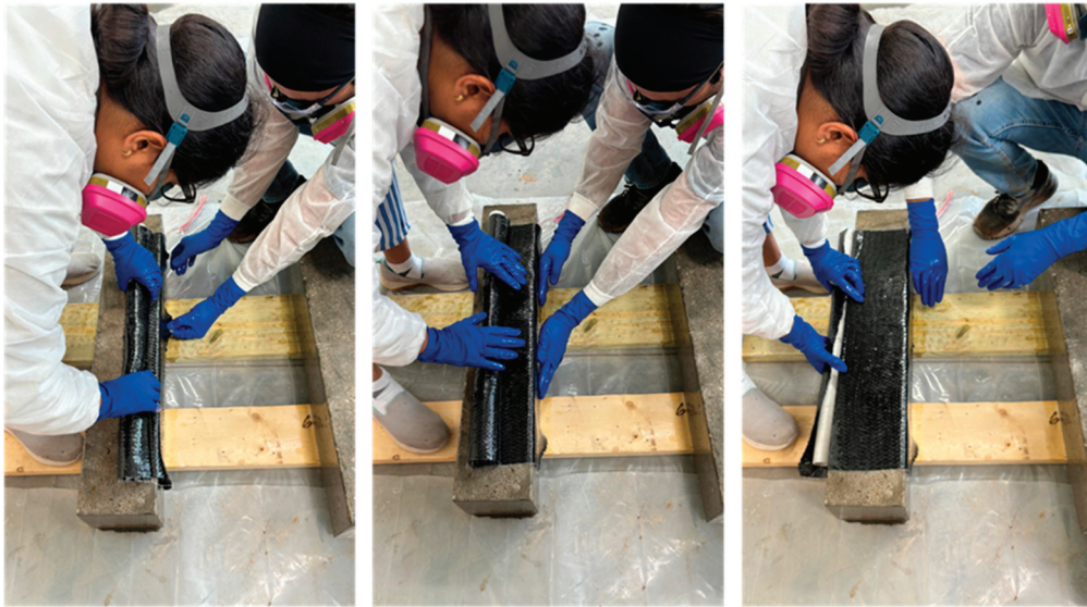
Figure 6. Rolling wet fabric onto pre-marked beam covering three sides for U-wrap.
