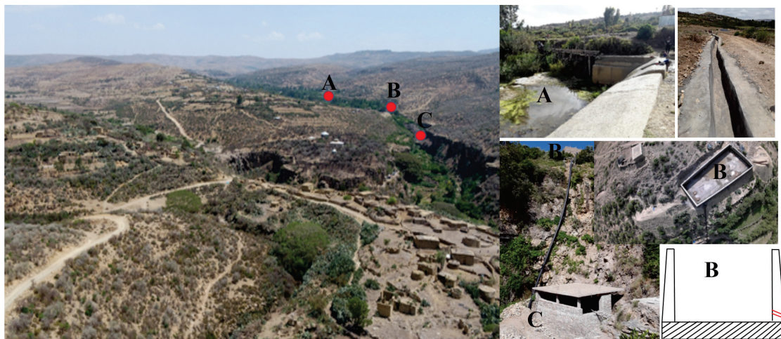
Figure 1. Amentila small hydro site: (A) diversion, (B) reservoir, and (C) powerhouse.
