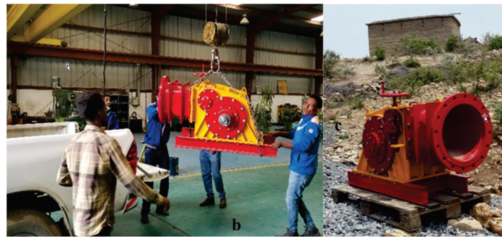
Figure 15. Finishing, receiving, and transportation: (a) prepared turbine at manufacturing company, (b) transportation to site, and (c) prepared turbine at installation site.
