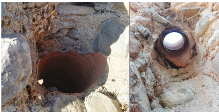
Figure 7. Amphorae deployed as air- and water-pipes in secondary use are found in both structures. (Photos: A. Tantsis).
