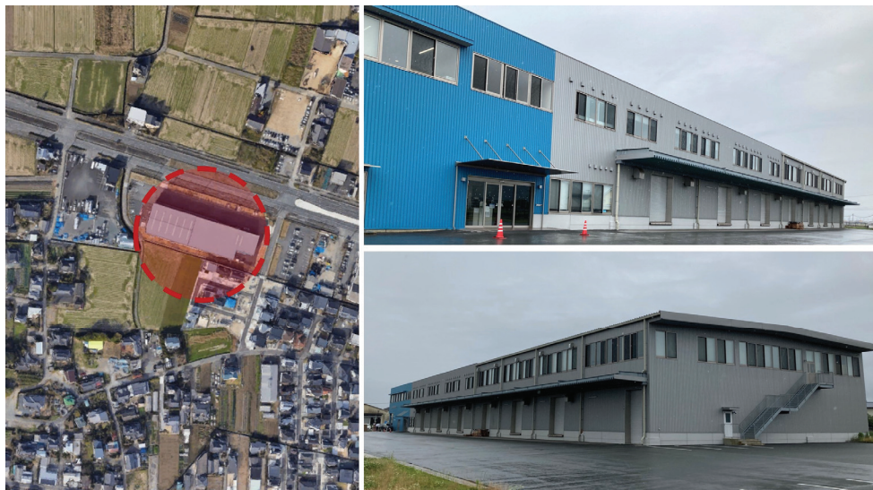
Figure 1. Building selected for the case study. The red dashed circle highlights the location of the Nori Distribution Center.
